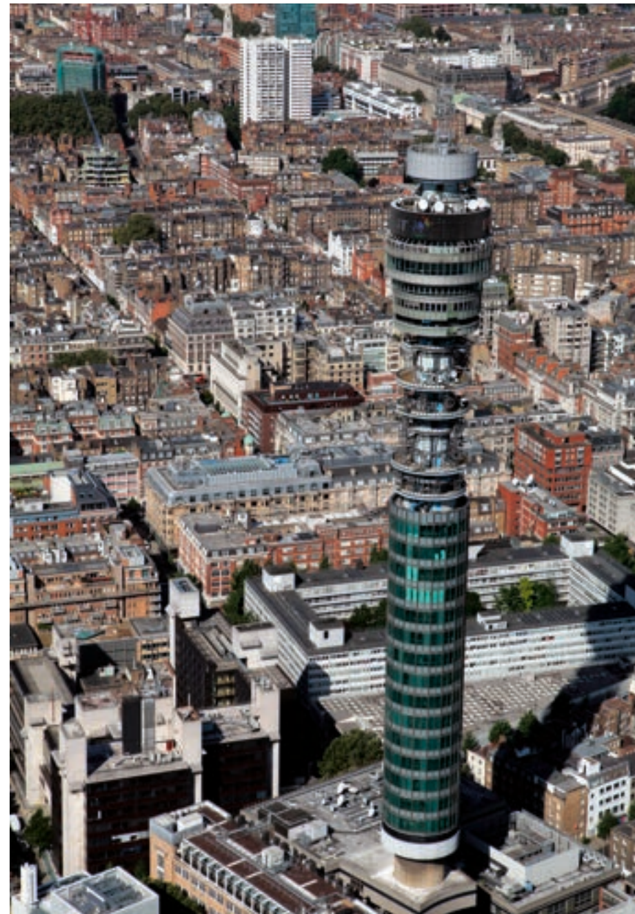
Belden supplies metallic cable products to British Telecom (BT), the largest provider of fixed-line, broadband and mobile services in the United Kingdom. Above, BT's iconic office tower in London.
