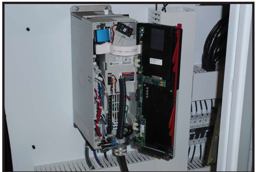
VFDs provide many advantages over single-speed motor control, but care must be taken with connections between the VFD and the motor.
