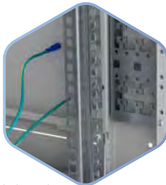
Lacing panel accessory installed
