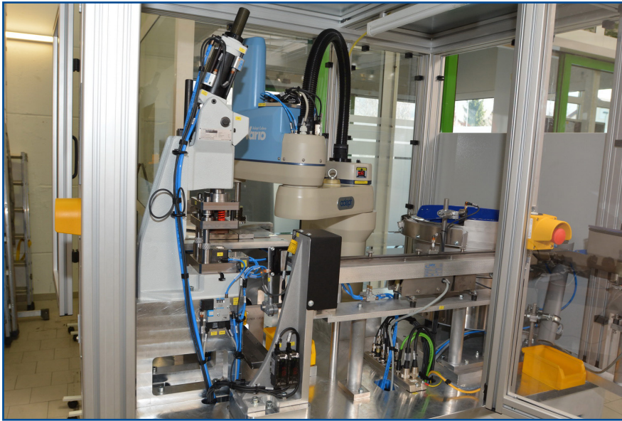
Multiple control signals in the robot cell ensure the precise measurement of thread thickness.
