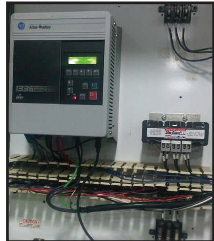
Variable frequency drives are increasingly used as a way to lower energy costs and increase the precision of a process control system.
