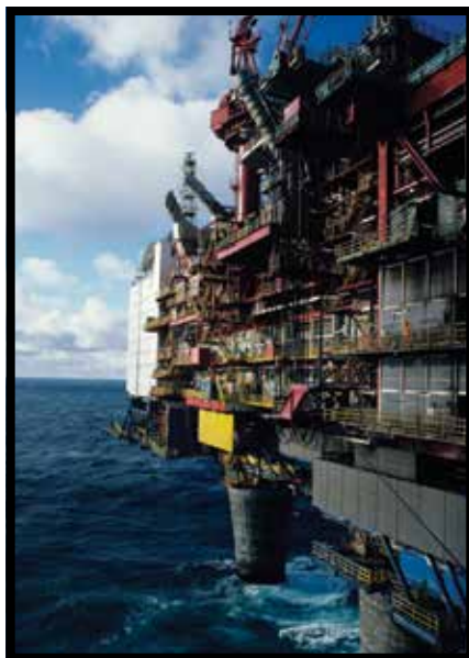
Natural gas and oil processing platform
