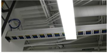
Belden's Small-Diameter 10GXS Category 6A Cables were used to ensure robust performance and support PoE LED lighting technology. The cable's size provides up to 25% space and weight savings, as well as easier installation. It also kept project timelines on track with easy-to-separate pairs and easy-to-remove barrier tape.
